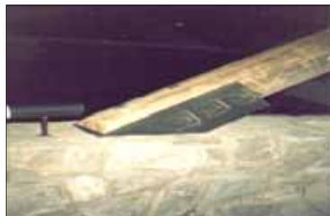
Timber Connection using a bolt
